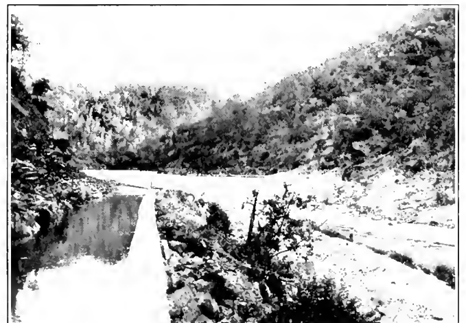
SOURCE OF WATER SUPPLY FOR FAIR OAKS AND VICINITY. DAM OF THE CALIFORNIA CORPORATION
